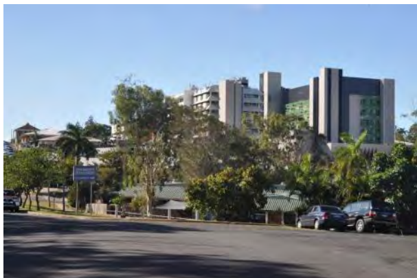
Photograph 2: Rockhampton Hospital March 2014 from Quarry and Cambridge St. corner.
