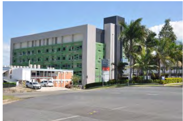
Photograph 3: New cancer services building viewed from the Canning St entrance to the hospital.
